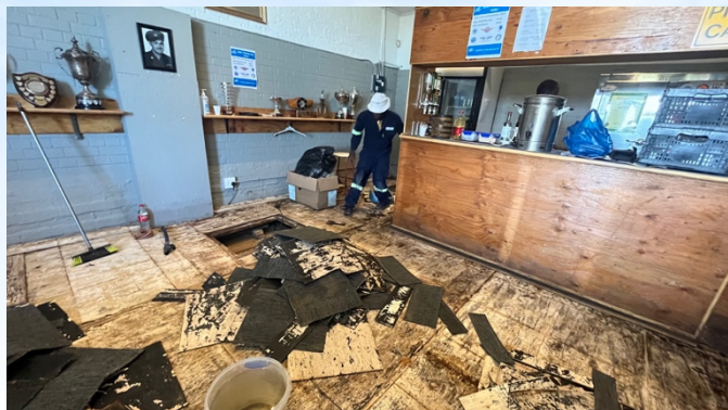
Stripping the old tiles from the bar area
