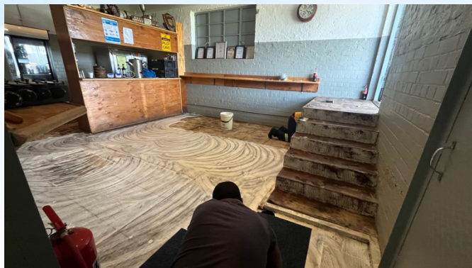
... glue down and ready for the new tiles!
