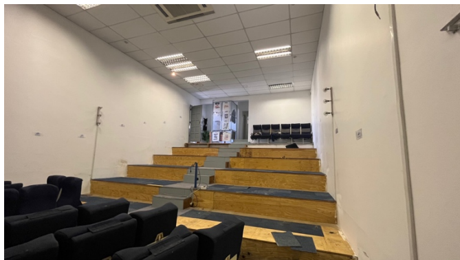
Seats out, ready for carpet replacement!
