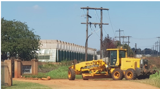
The Road Grader used to smooth the access roads
